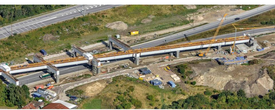
The bridge deck has now been casted and is ready for the rails, ballast electric lines etc.
