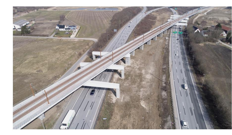
TP 30 crossing two motor roads in a skew angle.
