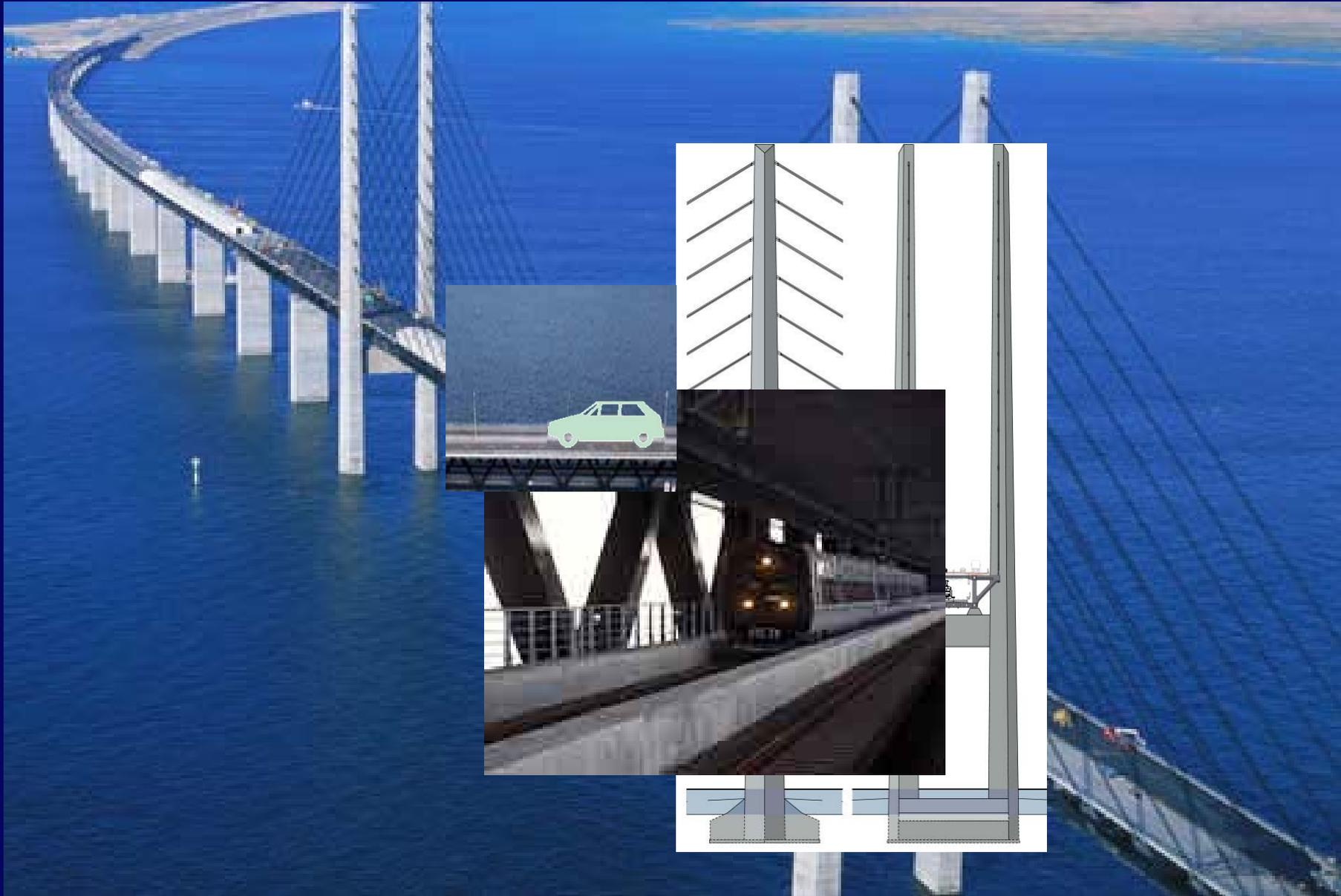
4 LANE MOTORWAY ON TOP OF TWO RAILWAY TRACKS
