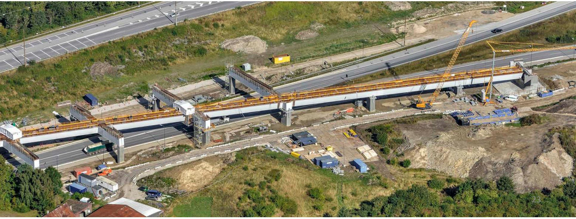
The bridge deck has now been casted and is ready for the rails, ballast electric lines etc.
