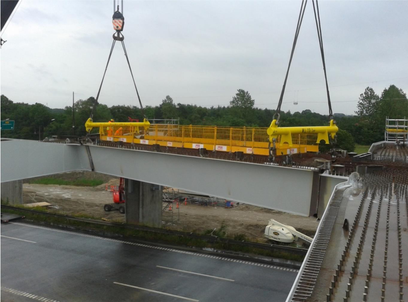
Provisional bolted joint between main girder and cross girder.
