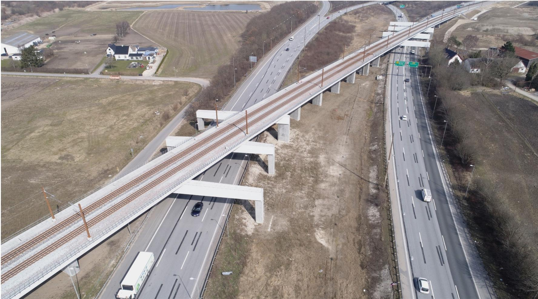
TP 30 crossing two motor roads in a skew angle.
