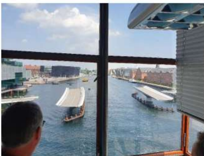
Bridge operated from control tower
